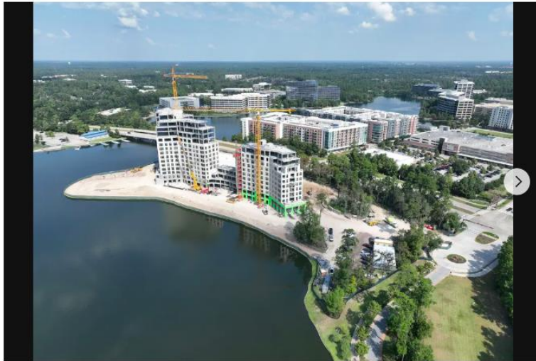
An Oct. 2, 2025 aerial image showing the Ritz-Carlton Residences, The Woodlands, an 111-unit luxury condo tower under construction near Lake Woodlands north of Houston. Courtesy of Howard Hughes Communities'
